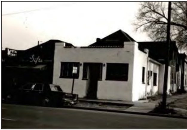
Figure 6. The dental office of Denver civil rights leader Dr. Clarence Holmes stood at the corner of Welton and 26 th streets until demolished recently for a large residential development. SOURCE: 2602 Welton Street, 5DV.76, survey photograph, 1981.
