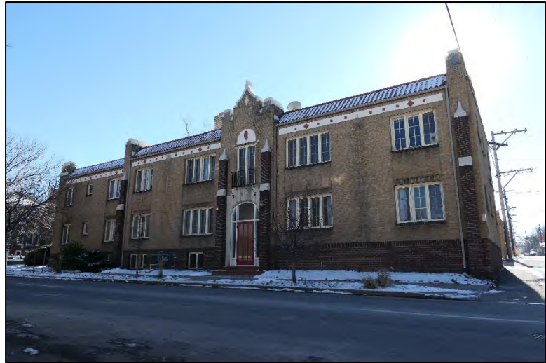
FIGURE 31: GERALD GERASH AND LYNN TAMLIN’S APARTMENT BUILDING AT 2330 E. 13 TH AVENUE IN DENVER’S CAPITOL HILL NEIGHBORHOOD. (AMY UNGER)
